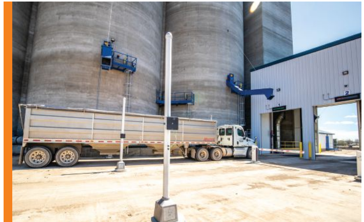
Tags mounted on grain trailers and RFID key cards are used at checkpoints to ensure grain is being delivered to the right dump pit and credited to the correct customer account. Systems are in place to call out inconsistent data.
